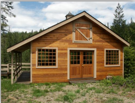
Rear of cabin
