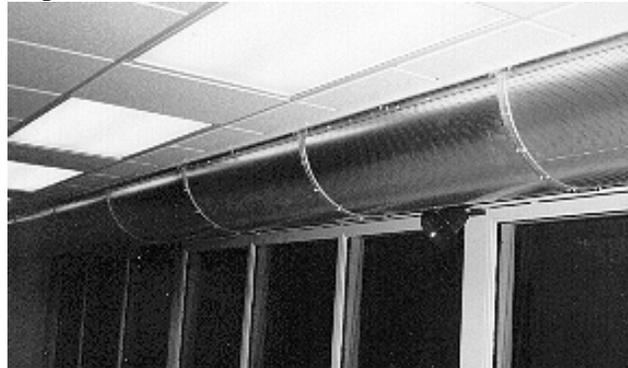
4.2.3 Dampers/diffusers. Many ranges have supply air distribution systems using dampers or diffusers. These are least desirable since they produce jets of air that can produce turbulence at the firing line. If diffusers are present, they should be located on the back wall behind the shooters. Diffusers should be sized to produce no more than 400 feet per minute maximum velocity.
