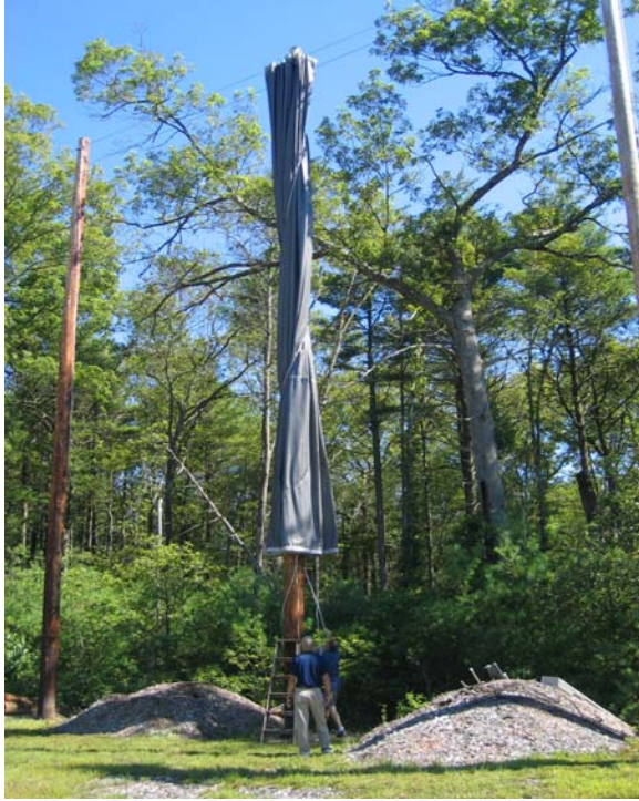
Figure 10: Photograph of Draw-Drape LSC Design Developed by the Standish Sportsmen's Association; LSC Deployed at SSA, East Bridgewater, MA
